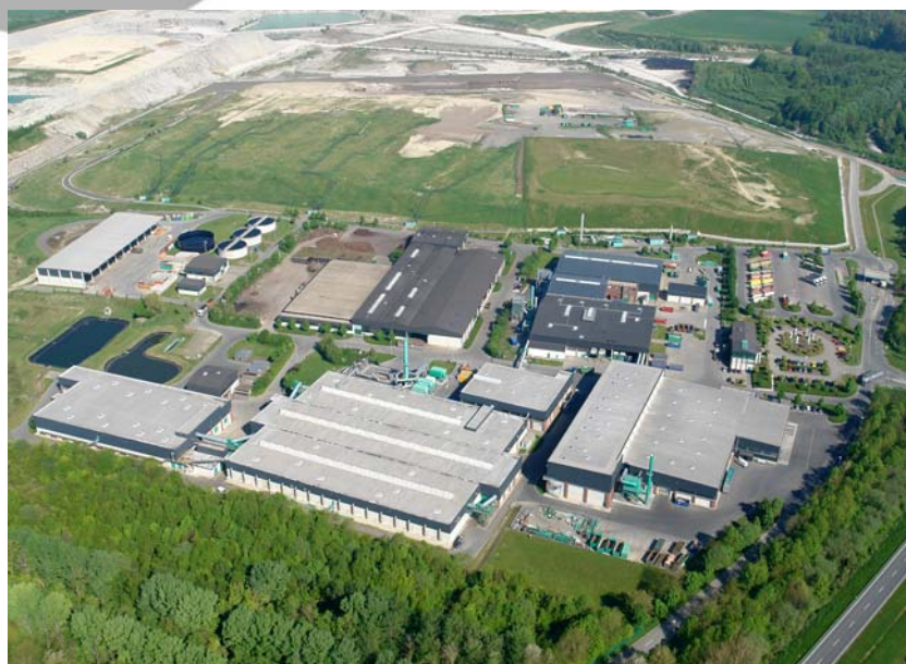
Bird's eye view of the Waste Management Centre in Ennigerloh
